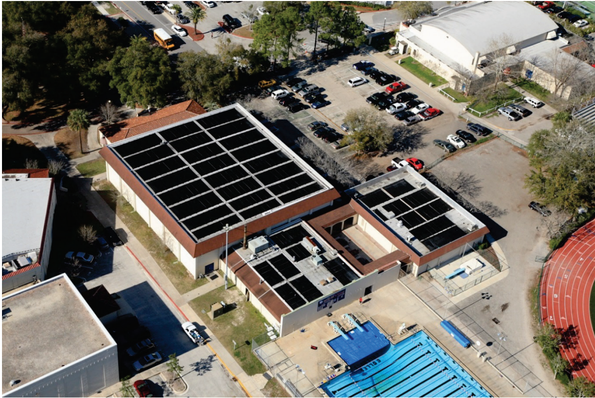
The Bolles School in Jacksonville, Florida has a 15 million BTU/day solar pool heating installation. (Photo: Solar Source)
