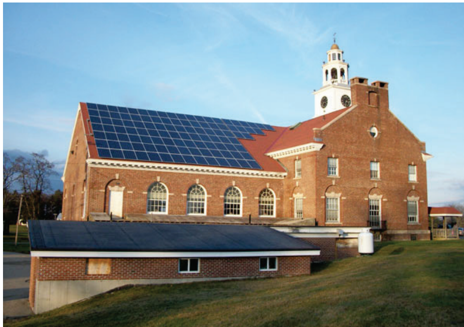
A 26 kW grid tied photovoltaic array for Good Will-Hinckley school in Hinckley, Maine, installed through a power purchase agreement. (Photo: ReVision Energy)
