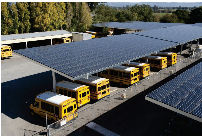
A 416 kW system at Analy High School in Sebastopol, CA. (Photo: SunPower)
